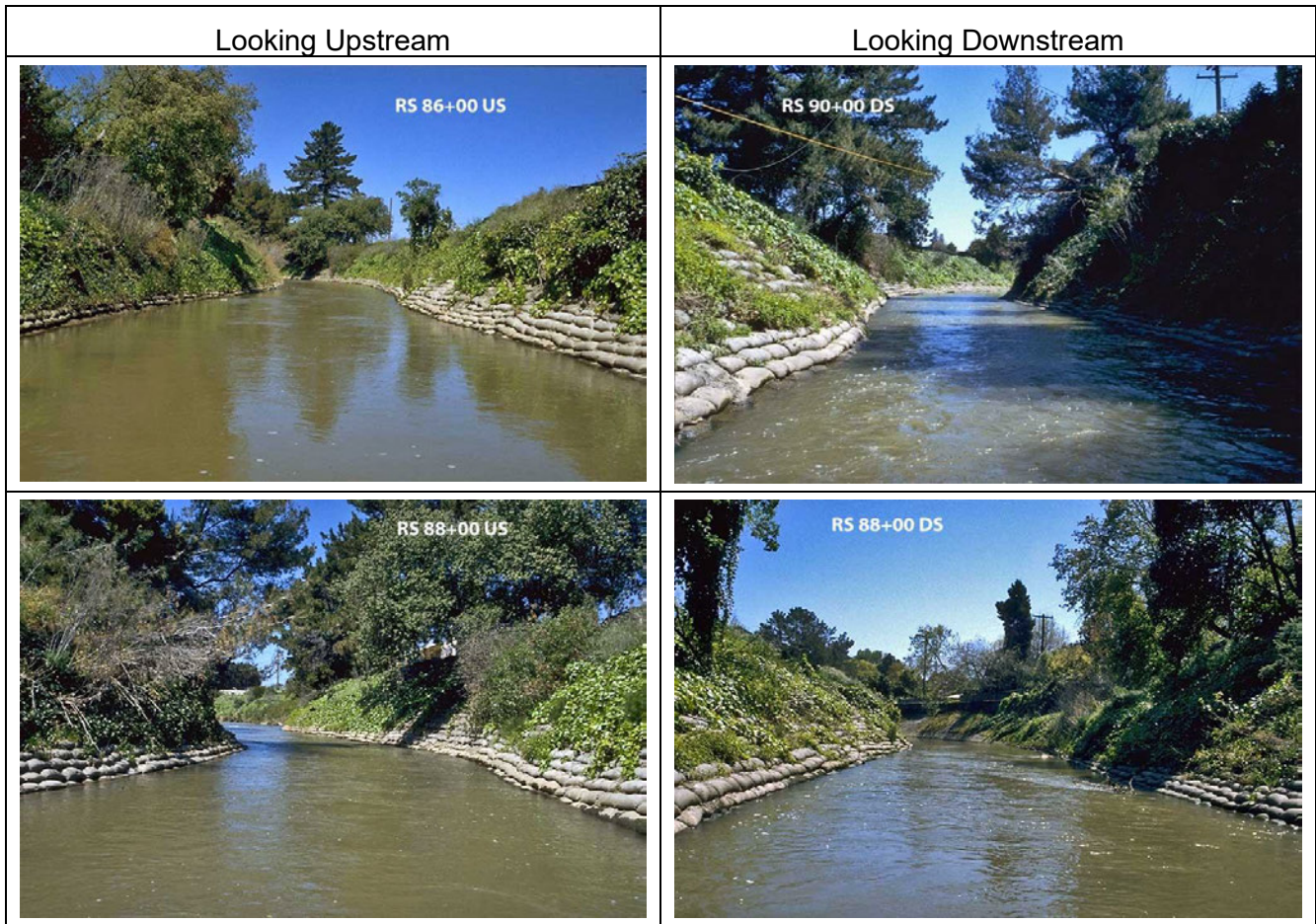
Figure 6: Upstream and Downstream SFCBS&R photographs of ~RS 87+00 to 89+00
